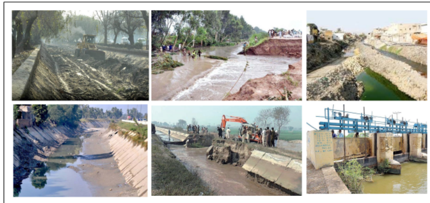
Figure 1-2: Top left: The process of silt removal accumulated at the Lahore Grand Canal is underway. Top middle: Water channel bank breach at Faiz Ganj canal due to flooding in Punjab, Pakistan. Top right: Effect on Liyari river due to the urbanization at the suburbs of Karachi, Pakistan. Bottom left: Shows accumulation silt at one of the canals in Punjab, Pakistan. Bottom middle: A brick-lined canal is breached 60 feet wide at the Jhang Branch canal due to lack of maintenance. Bottom right: Shows a wearing structure of a canal head in Punjab, Pakistan.
