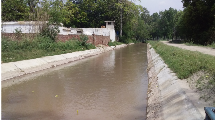
Figure 6-2: The experimental Raiwind- 1 canal view with uniform and paved structure.
