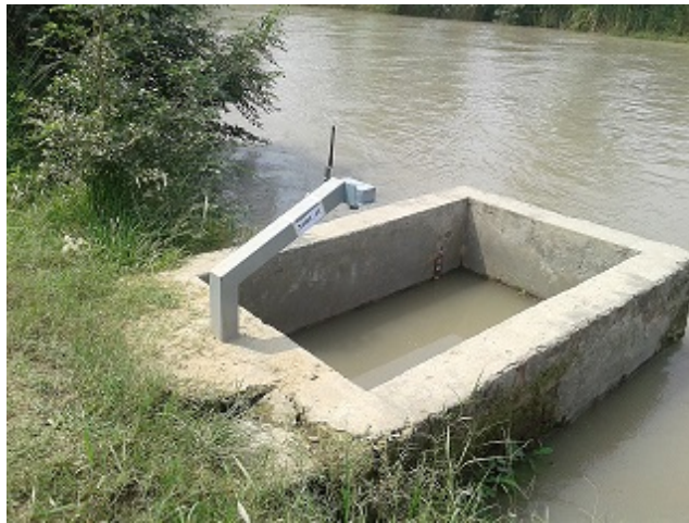
Figure 3-2: Eulerian sensor providing the data of water level in canal.
