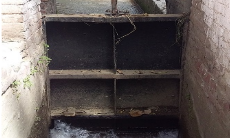
Figure 6-4: The undershot gate at the start of canal to control the water flow in canal and provide boundary condition values.
